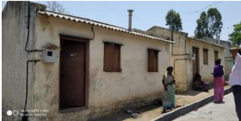
Houses constructed for relocated Jenu Kuruba families from Nagarhole National Park
